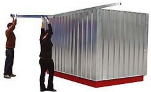
6. Slide the roof on top of the building
