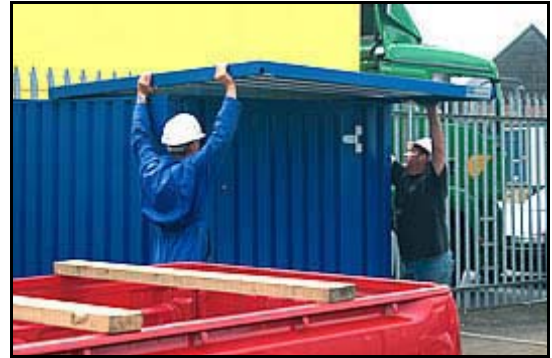
Lift on and fix the roof in place
