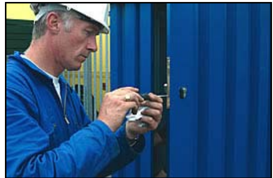
Install the door locks
