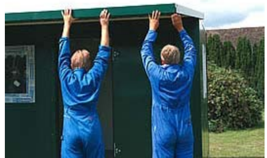
Fit the outer roof skin
