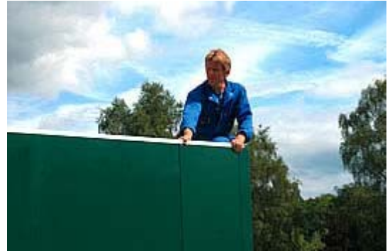
Fit the ceiling retention bars
