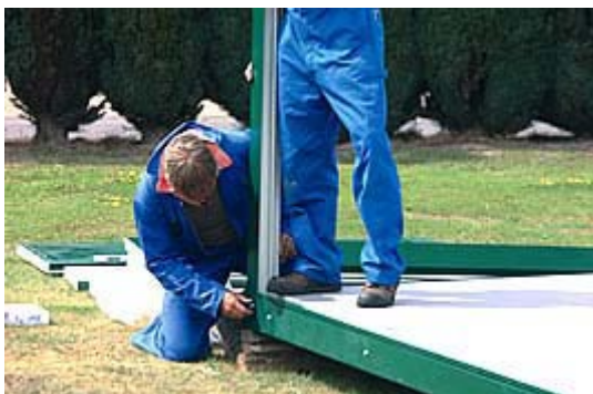
Fix the four corner posts
