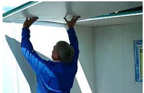
Slide in the ceiling panels
