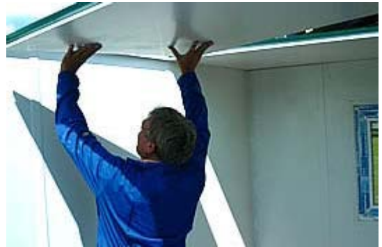
Slide in the ceiling panels
