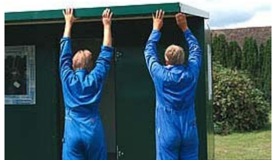
Fit the outer roof skin
