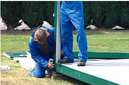
Fix the four corner posts
