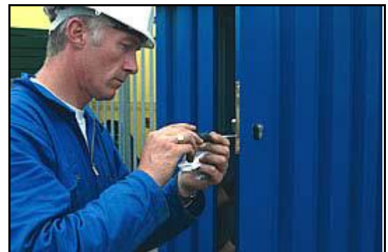
Install the door locks
