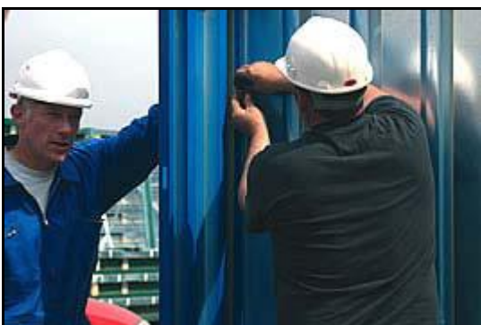
Fix the holding screws
